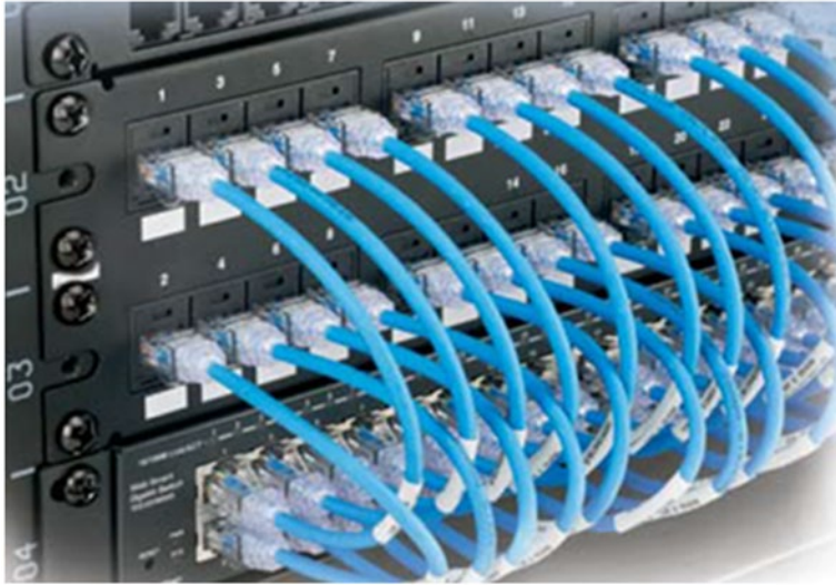
Example of one-to-one switch patching
