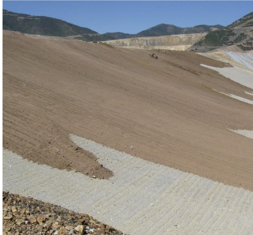
Left: Relaxed slope; Right: Cross-ripping and soil; 2008-2012 dump rehab
