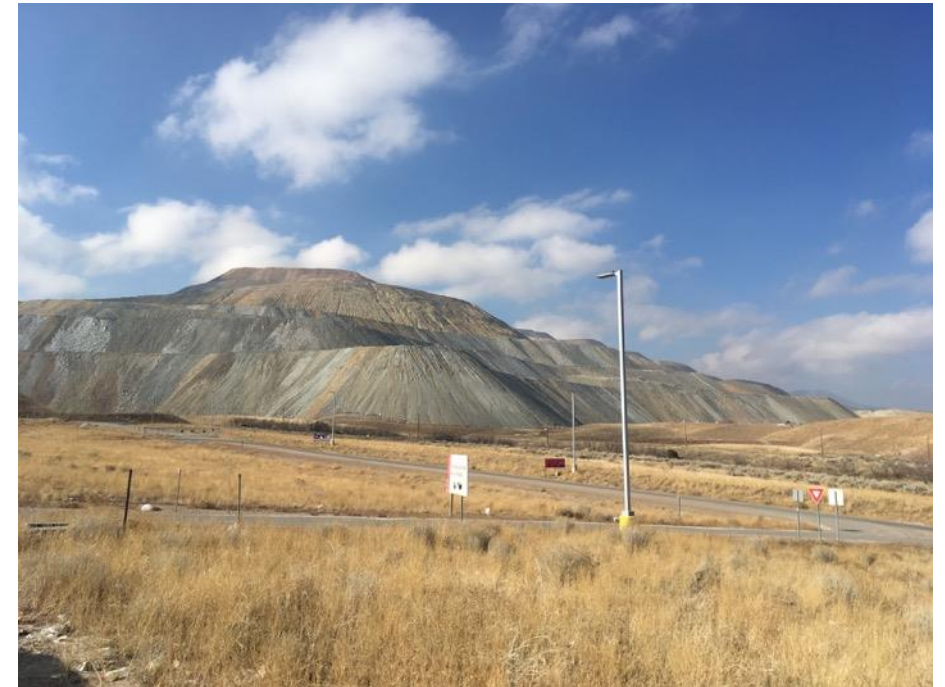
Phase I slopes regraded 2.5:1
