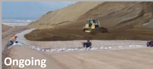
Barneys Heap Leach Area
