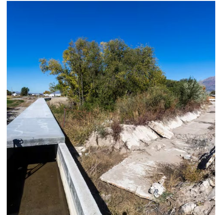
Canal infrastructure replacement reduces water loss to evaporation. Image Credit: Brian Nicholson.
