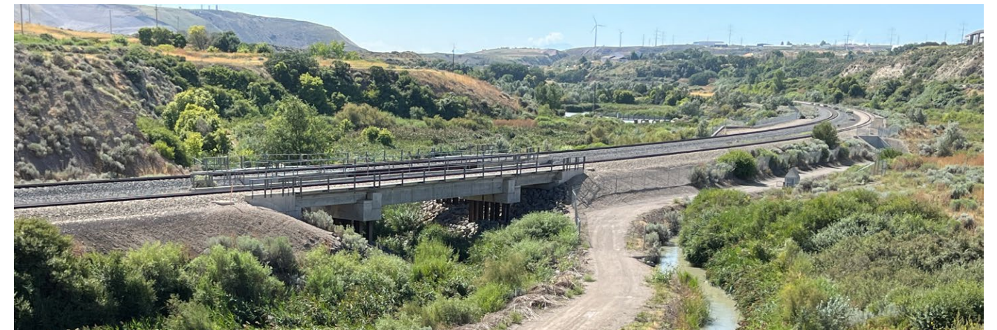
The Jordan River near the confluence with Beef Hollow Creek and Wood Hollow Creek
