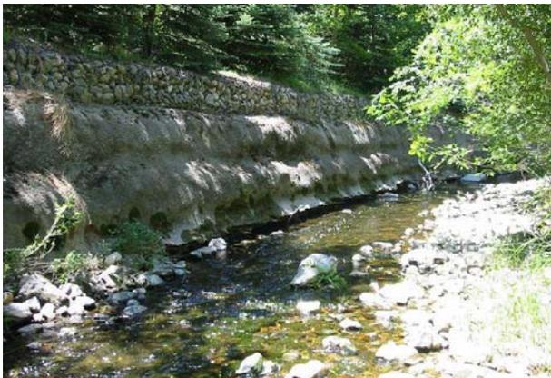
Many improvements to Big Cottonwood Creek occurred in response to flooding in the mid 1980s. Gabions (pictured here with a concrete covering) were used to protect banks from erosion. In addition, the Old Mill debris basin was constructed to reduce sediment and tree branches from moving downstream and blocking culverts causing flooding. New techniques of restoring habitat as well as protecting banks from erosion are now encouraged as a BMP and an alternative to gabions (see Figure 18 on page 22.)
