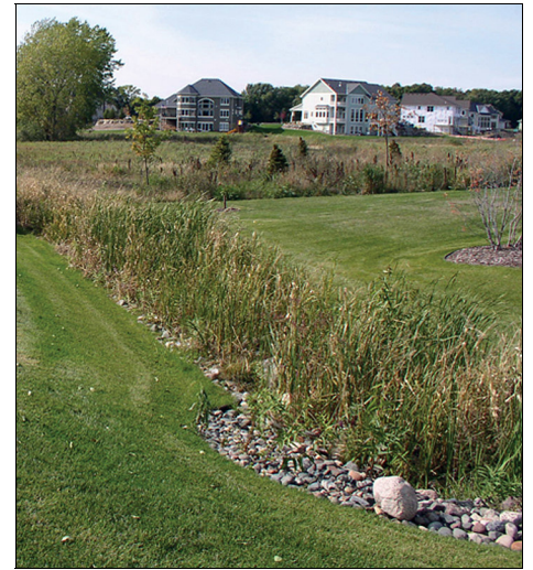
Example of a bioswale, a vegetated channel that conveys stormwater runoff while slowing down the flow. This allows sediments and pollutants to drop out, and water to infiltrate back into the soil.
