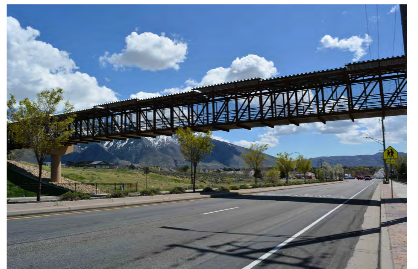
EXAMPLE OF VERY SIMILAR BRIDGE
